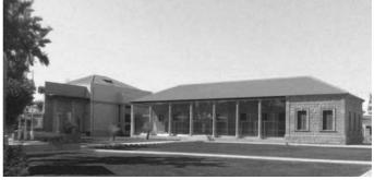
system (geothermal heat pumps), lighting and glazing. Double glazing on north and east sides, laminated glazing on west side. The walls remained indoor and outdoor limestone, but the internal wall was insulated with polyurethane foam. A solar chimney was built for preheating the air.
