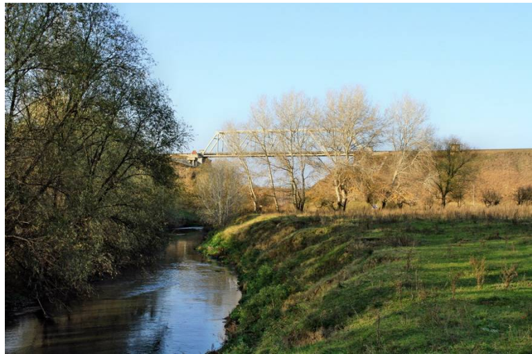
Figure 1: Bâc River (near Calfa Village) a typical medium river, Source: Dr. Ilya Trombitki, Eco Tiras
